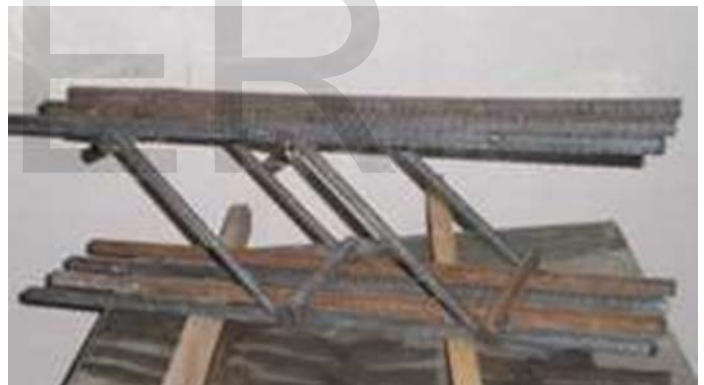
Fig. 1: Typical welded swimmer bars
